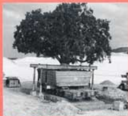
12 Relocation live oak tree in California
